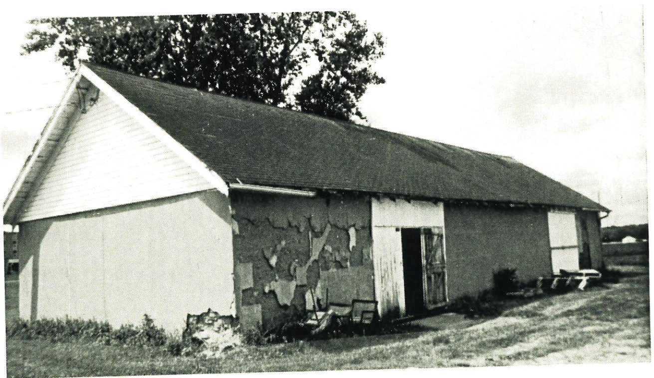
Figure 4-Experimental Rammed Earth Machine Shed
